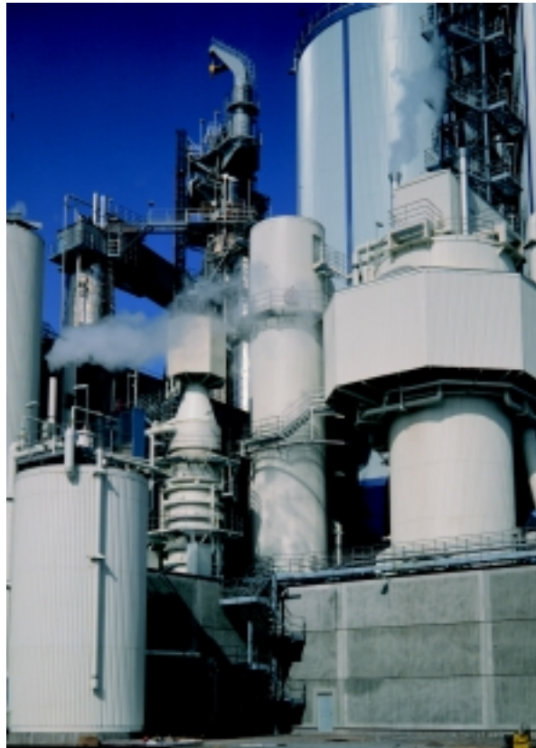
Skoghall, Sweden, O 2 plant
