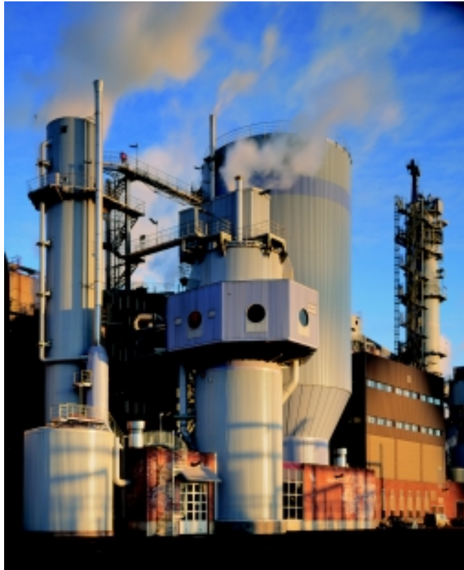
Kymmene mill, Finland, O 2 plant
