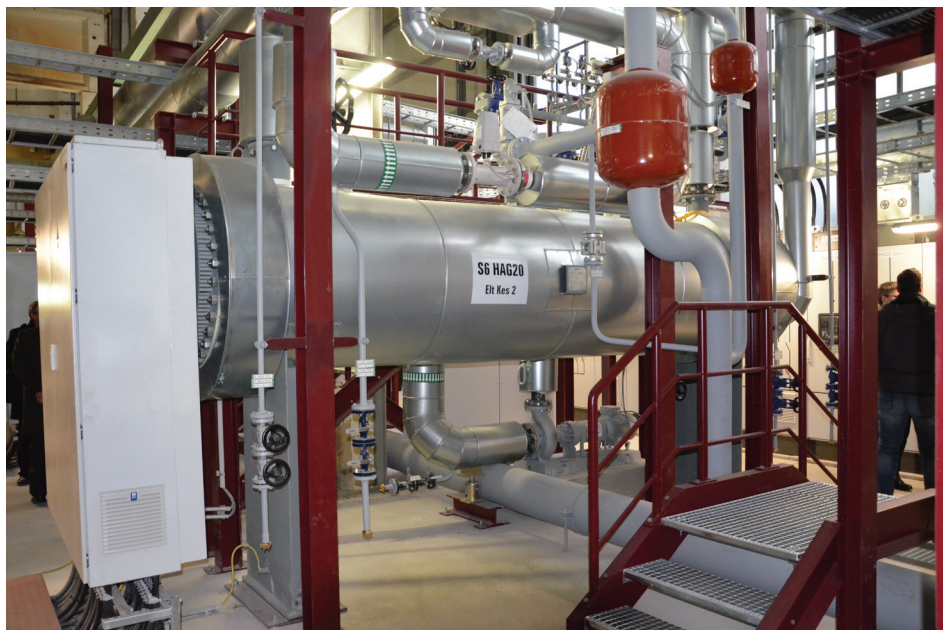
Figure 2. A 5 MW boiler power-to-heat system at the municipal utility of Schwerin with 250 heating elements that are subdivided into 14 heating groups (Source: Klöpper-Therm)
