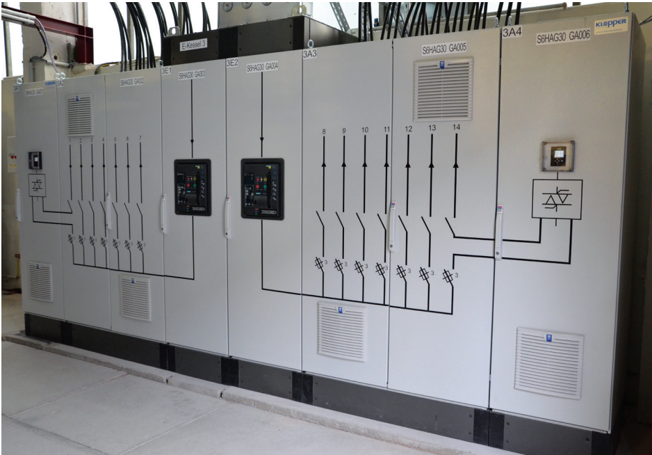
Figure 3. Power supply for power-to-heat at the municipal utility of Schwerin for a 5 MW boiler with two Thyro-P 2P690-500HF power controllers and a Thyro-Step Controller for 2x7 heating circuits (Source: Klöpper-Therm)
