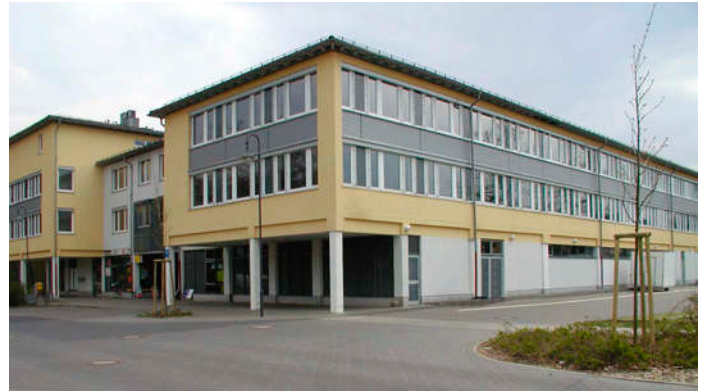
Allectra GmbH facility near Berlin (Germany)
