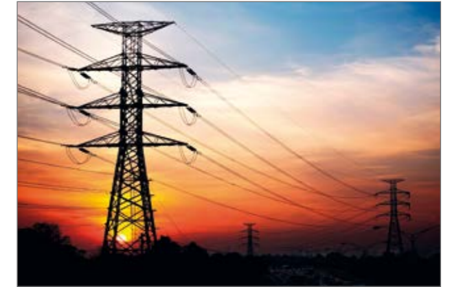
Power distribution and industrial automation
