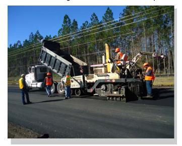
•The mix was placed ~100°F lower than the standard mix with no reduction in density and Marathon was extremely happy.
