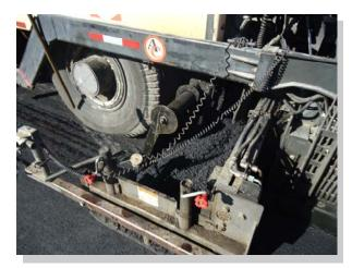
Mix was workable in areas where hand work was needed. Paving crew comments where that the mix did not feel "heavy" as traditional hot mix usually becomes when hand work is required. Comments were made by the paving crew about less smoke and fumes as compared to traditional hot mix.
