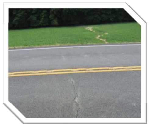
After 10 months, the control section has cracked while the PMAE section has not cracked
