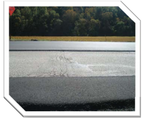
The upper lane has already been paved and the unpaved section is the general condition of the transverse cracks before BondTekk application
