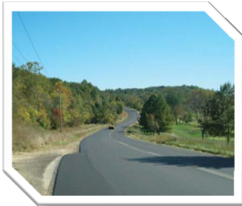
Missouri Route T with BondTekk application complete
