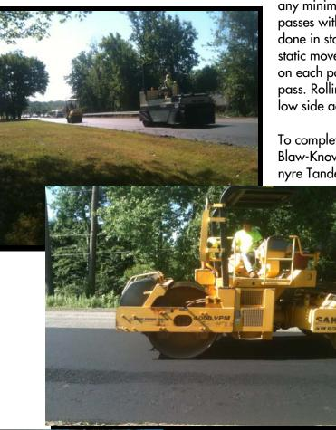
any minimum density requirements. All rolling passes with the breakdown and finish rollers were done in static mode. The pattern consisted of one static movement up and one static movement back on each pass before moving over to start the next pass. Rolling was done from the high side to the low side across the mat.
