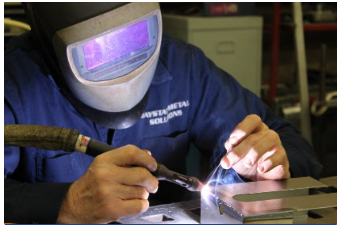
Welded components require precise joining utilizing MIG, TIG or other forms of welding.
