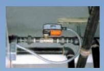
Characterized Control<sup>™</sup> Valve (CCV) with LF Series Spring Return Actuator.
