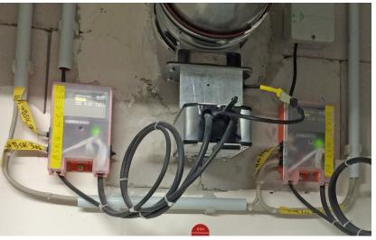
Each of the 900 fire damper actuators installed at the Hamm-Lippstadt University of Applied Sciences are controlled and monitored by a BKN230-24-MOD from Belimo. This ensures that the status and possible malfunctions of the fire dampers are permanently visible, not only on-site at the device but also on the monitor at the operations centre.
