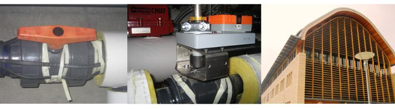
actuator on a PVC or any other type of valve. Traditionally control valves are metal, however with Belimo's new linkages, PVC was not a determining factor. Although Belimo has supplied special linkage kits for globe and butterfly valves for several years, this was the first ball valve retrofit kit. In fact, Kroon Hall, would become only the 3rd facility to use the ball valve retrofit kit.
