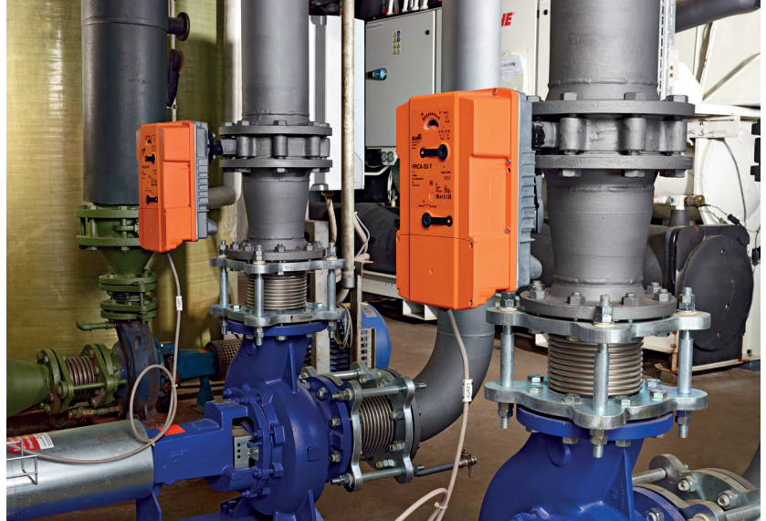
The innovative PR actuator installed in the new plant of Kuhn Champignon AG.
