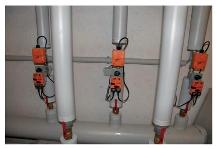
Each of the 14 heating circuits is equipped with a Belimo electronic pressure-independent characterised control valve (EPIV), which regulates the correct water quantity for each con-
