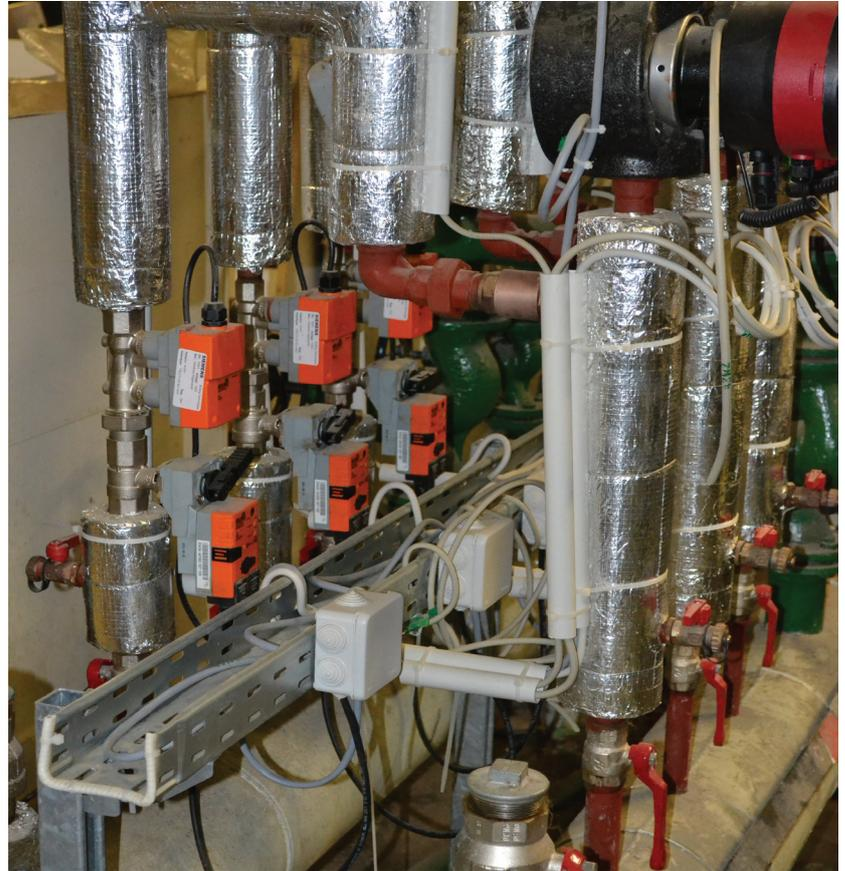
A total of 45 EPIV were fitted on eight distributors during ongoing operation. This wasn't a problem for Belimo's characterised control valve, which dynamically regulates hydraulic balancing.
