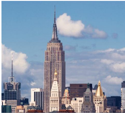
Empire State Building, NY
