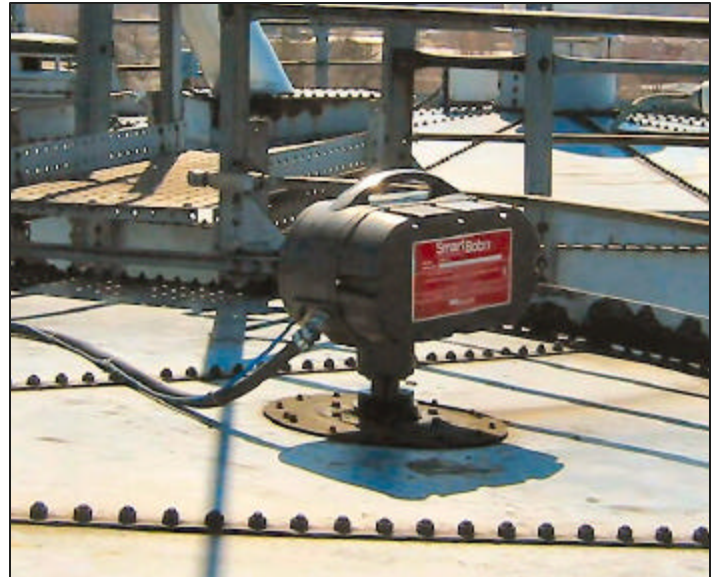
SmartBob II remote installed on roof of a 33 ft. Carbon Black storage silo at Goodyear
