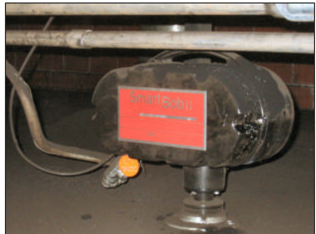
SmartBob II remotes are installed under a conveyor belt that sends coal into large storage bunkers that the units monitor
