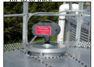
SmartBob II remote installed on the hatch of a polystyrene storage silo
