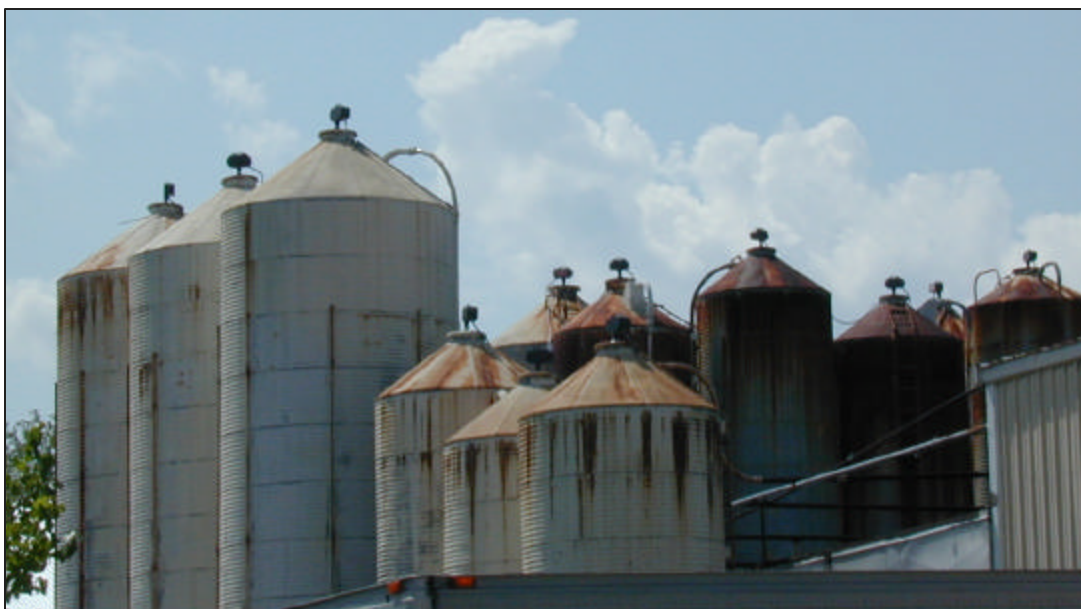
SmartBob II remotes measuring crystal polystyrene on outdoor storage silos at American Polymers
