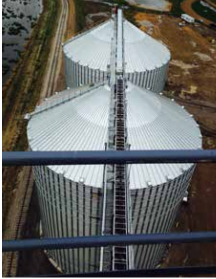
View of the new GSI tanks from atop the Bucyrus terminal's concrete workhouse.
