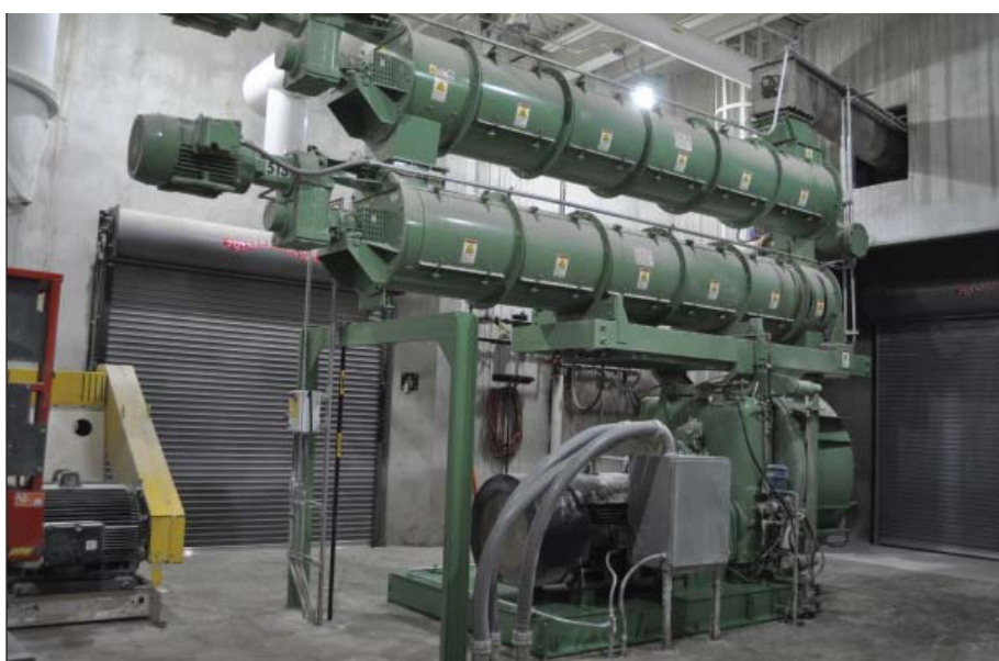
One of two CPM 600-hp pellet mills outfitted with dual CPM steam conditioners.
