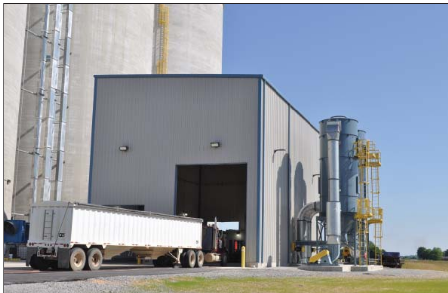
Two enclosed truck receiving pits, one of which doubles as a rail pit, are serviced by a heavy-duty Aircon baghouse filter at right.
