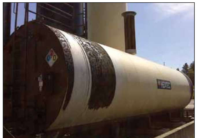
Horizontal Tank at Asphalt Plant
