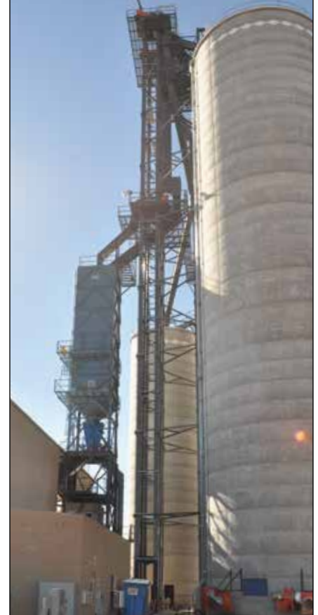
Grain handling equipment includes a pair of 30,000-bph Schlegel receiving legs, a 60,000-bph Schlegel loadout leg, and a 60,000-bph C&A bulk weigh loadout scale.
