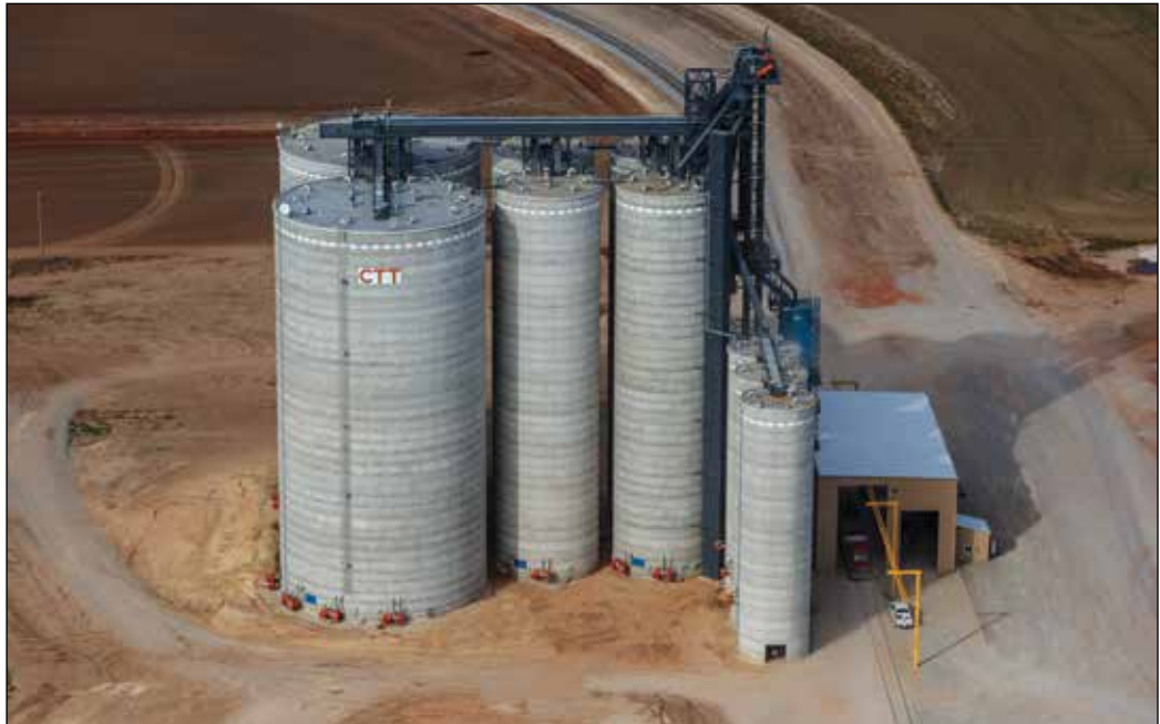
The new Chisholm Trail Terminal outside of Medford, OK, operated by Farmers Grain Co., features 1.5 million bushels of upright storage and 60,000 bph of receiving and loadout capacity. Aerial photo courtesy of McPherson Concrete Storage Systems.
