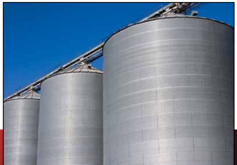
Large grain storage silos can be accurately measured.
