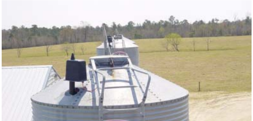
SmartBob-TS1 sensors measuring dry feed in eight 20' feed silos on a hog farm in Roseboro, North Carolina
