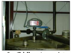
SmartBob II remote measuring mineral oil on an indoor liquid tank
