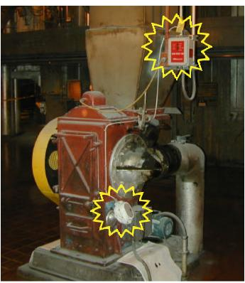
BinMaster Flow Detect 1000 mounted on a coal feeder at OPPD's North Station coal fired power plant in Omaha, Nebraska
