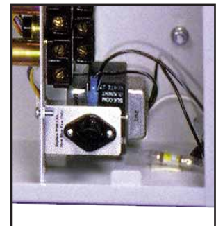
LP-2500/2600 Transformer and Fuse
