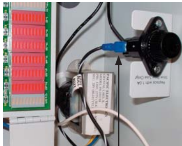
spade connector on voltage quick connect between transformer and fuse
