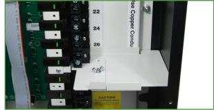
Reinstall LTR. DO NOT exceed 5 in-lbs when tightening LTR fastener.
