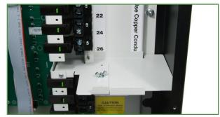
Insert Outside Divider. Mate threaded stud and alignment dowels with corresponding holes in Inside Divider. Install and tighten Wing Nut on threaded stud.
