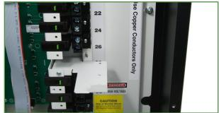
Insert Inside Divider and secure with Inside Divider Fastener. DO NOT exceed 5 in-lbs when tightening.
