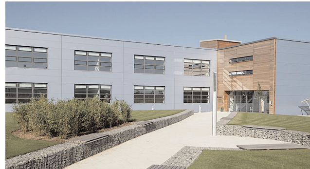
Oxford NanoLabs is based in the new purpose-built facility in Oxford, UK
