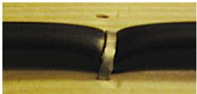
Figure 4.4b – ClearCurve Rugged Drop Cable Stapled to Joist | Photo NS162
