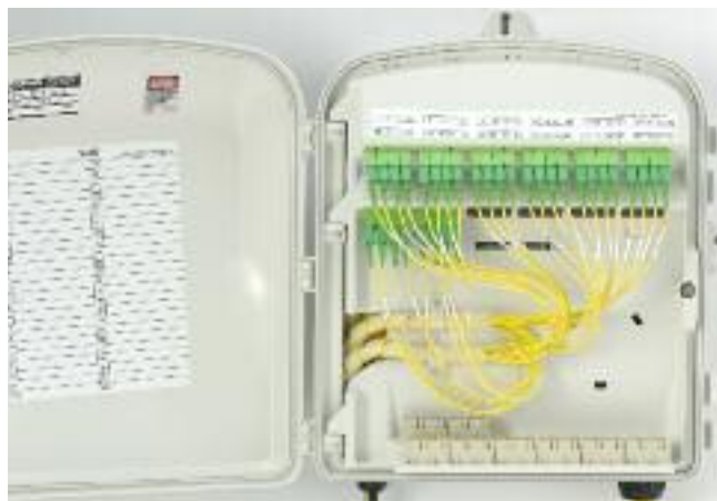
Figure 4.22 – OptiSheath MDU Splitter Terminal | Photo SHD213
