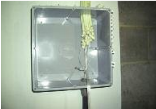
Figure 4.9 – Transition Pull Box | Photo NS122
