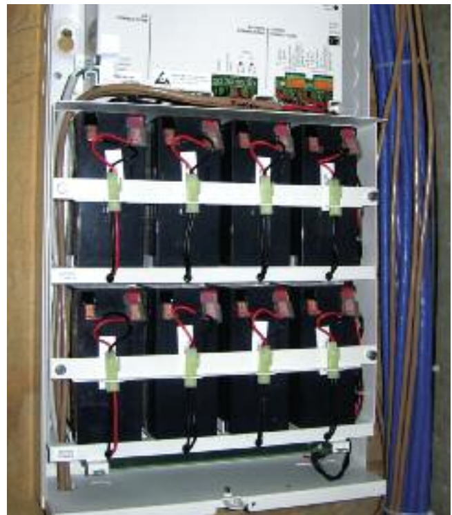
Figure 2.13 – Battery Backup for mu-ONT | Photo NS149
