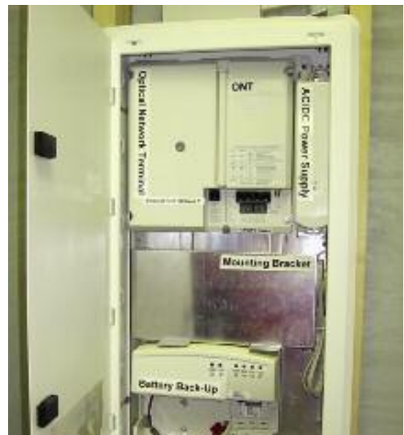
Figure 2.9 – ONT for Mounting Between Studs | Photo NS117
