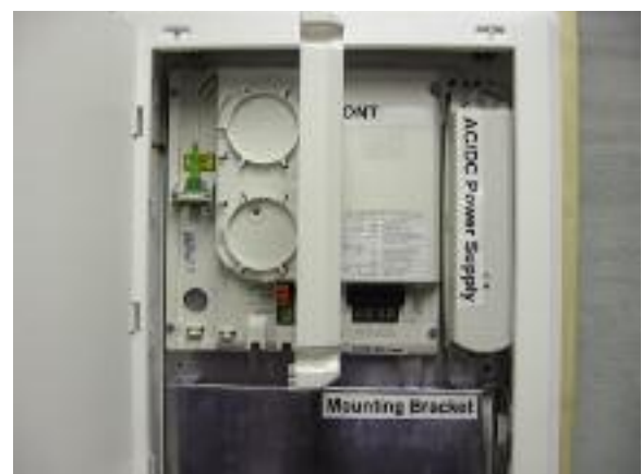
Figure 2.8 – ONT for Mounting Between Studs | Photo NS116
