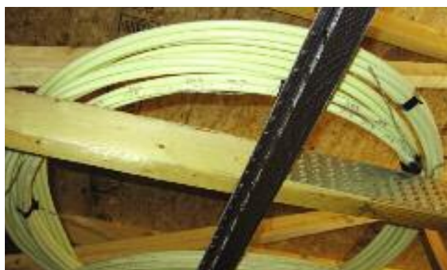
Figure 4.8c – Microduct | Photo NS121
