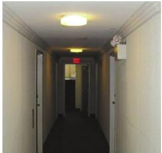
Figure 4.11 – Raceway in the Form of Decorative Crown Molding | Photo NS124
