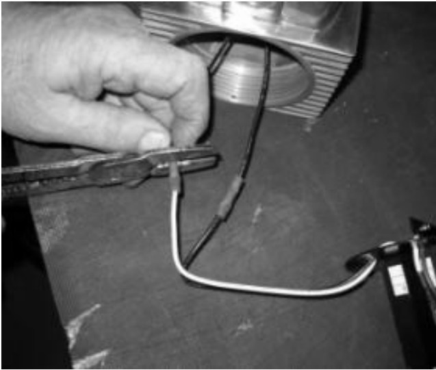
ATTACH LIGHT ENGINE USING CRIMP-TIGHT WIRE CONNECTORS [FIGURE 5]
