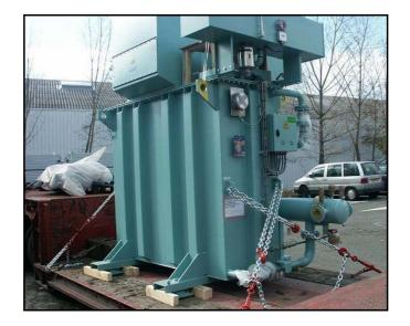
The unit must be on a wooden floor and rest on the substructures only. It must be carefully shored in both directions using wooden parts applied against the substructures. It must be securely slinged by lifting rings so as to seat it firmly on the floor and prevent it from tilting.
