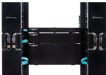
Ready 1U, 2U, 4U Shelves installed (closed)
