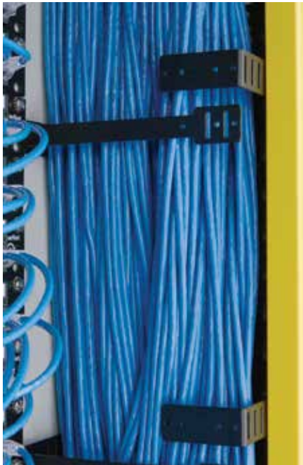
Vertical routing at 50% to 60% of capacity
