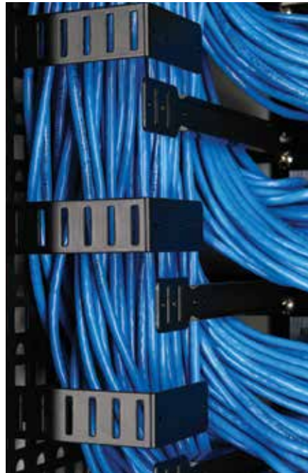
Horizontal to vertical transition at 50% to 60% of capacity
