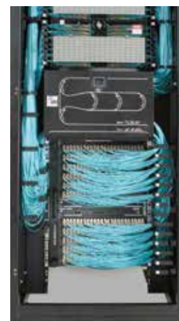
In-cabinet slack storage
