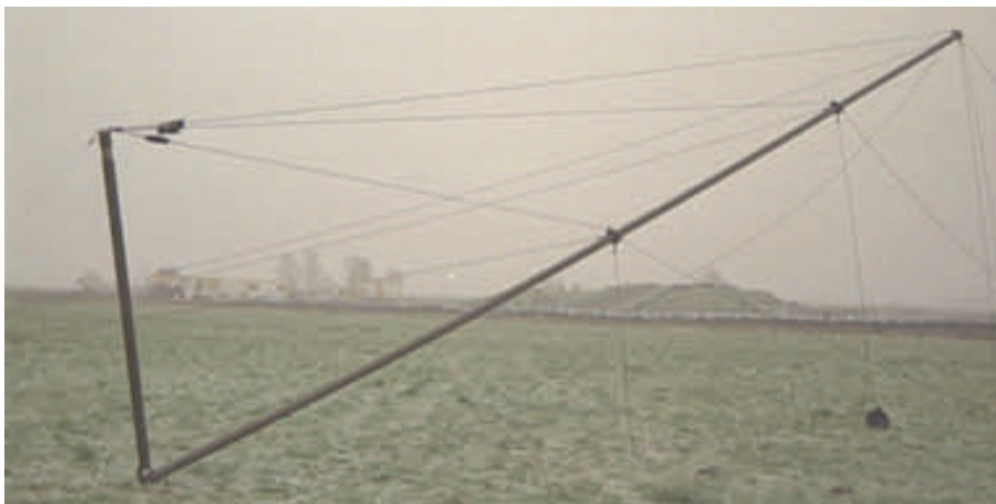
Tilting of a 15m mast
