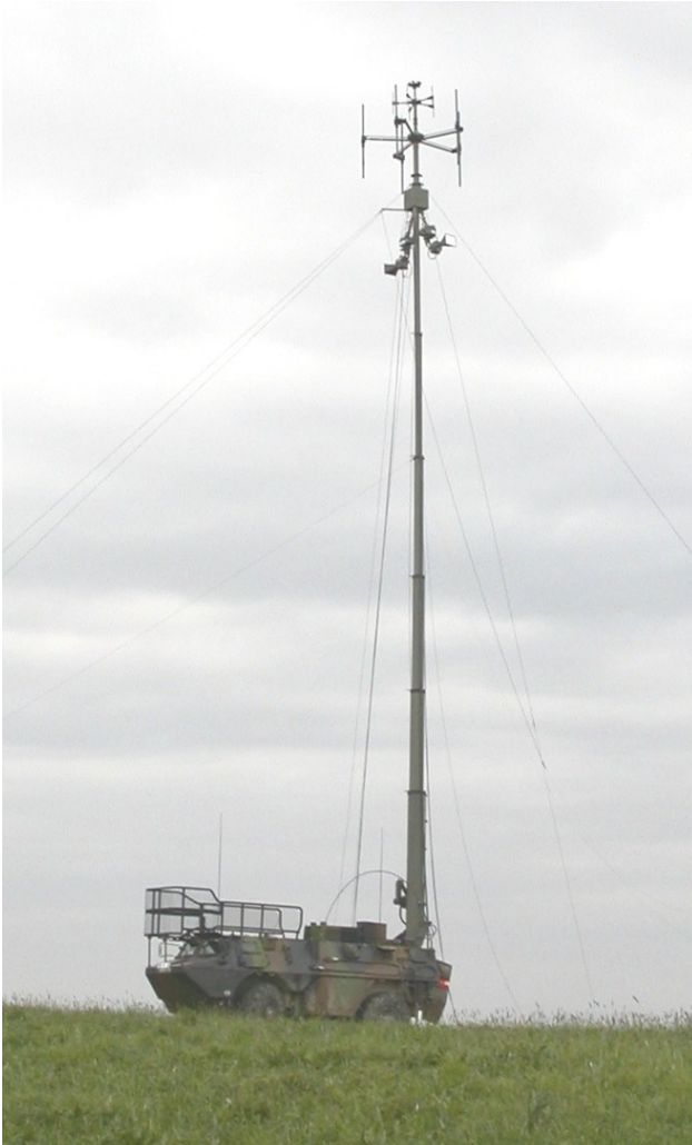
Mast fully elevated with guy lines
