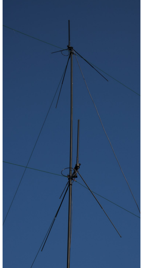
15 meter ULM-C 48/15-1.3 mast supporting Two Comrod VHF302000TB-TRI/TB-S elevated tri-band antennas
