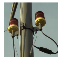
Night warning beacon
