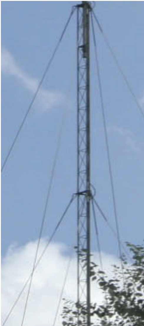
H100 used to guy a lattice tower
