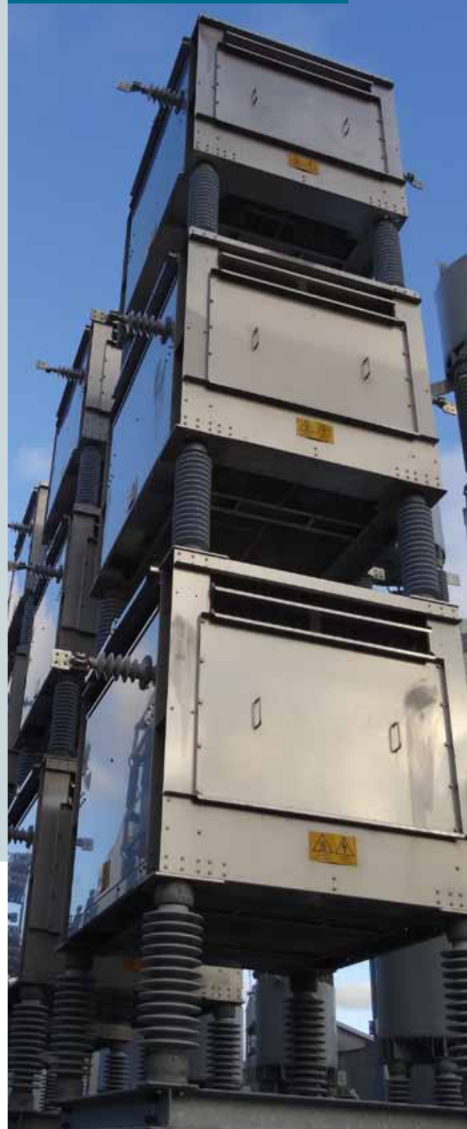
Resistors operating as part of an SVC network in an Aluminium Smelting plant in Canada.
