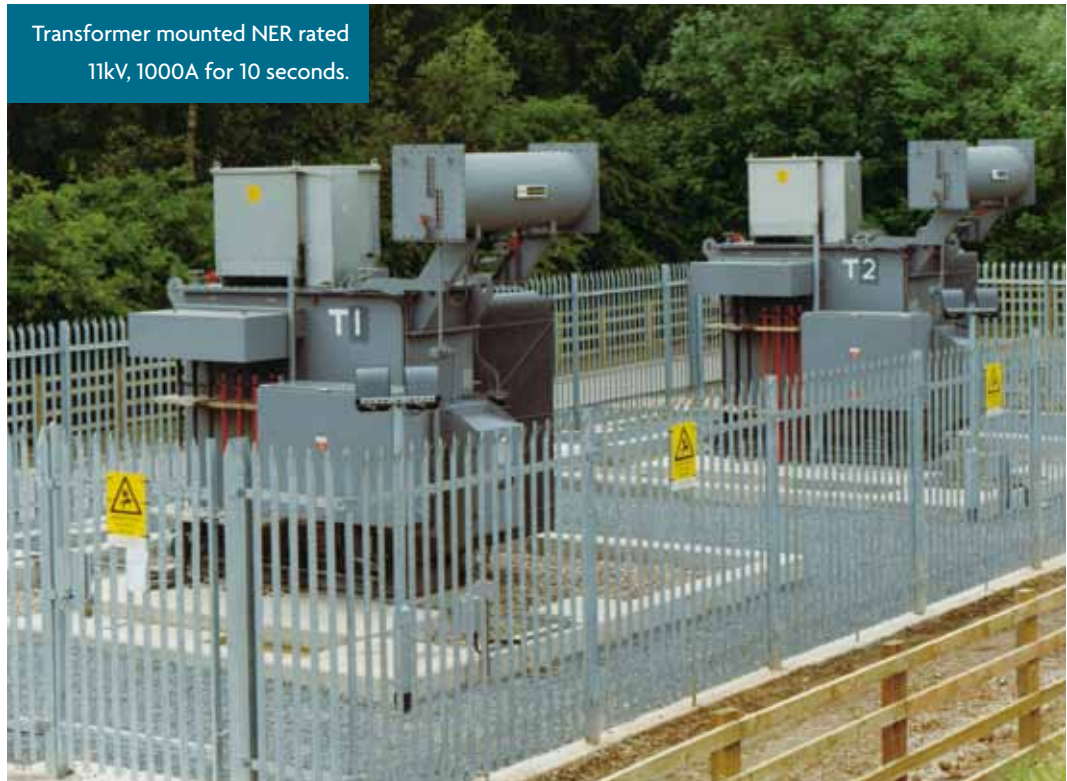
NER and vacuum contactor assembly in a UK Utility substation.
