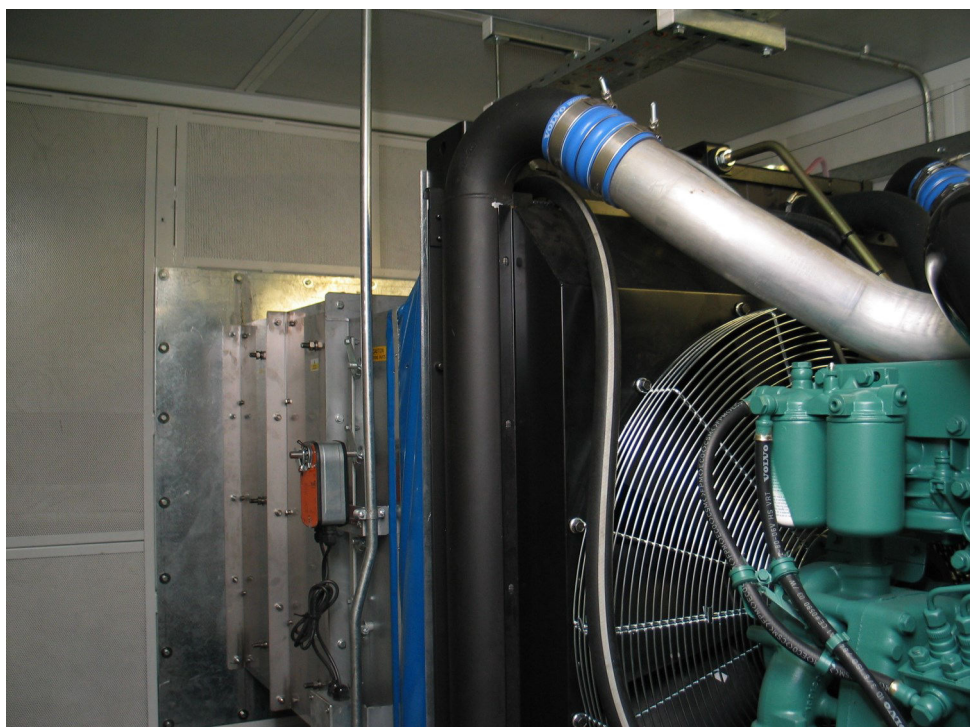
In some cases, the same load bank can be used as a ballast load during normal operation of the generating set.
