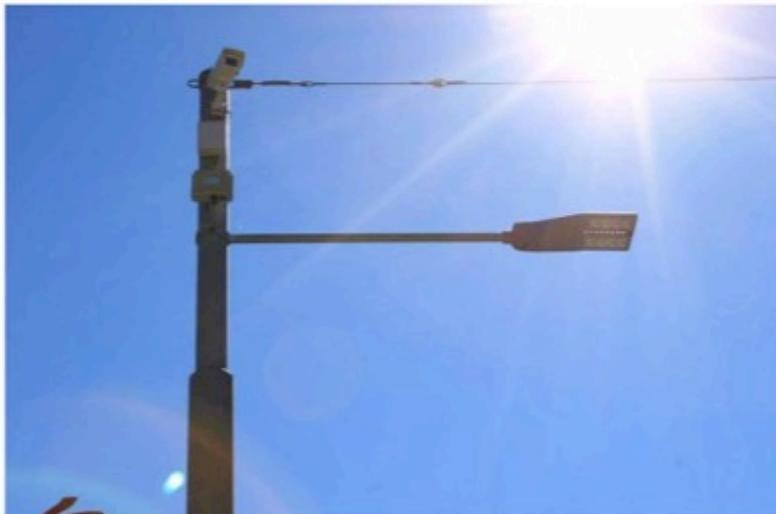
*IP cameras are installed on light poles, taking advantage of PE.AMI network infrastructure*
