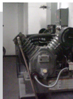
Air Compressor – Full Visible
