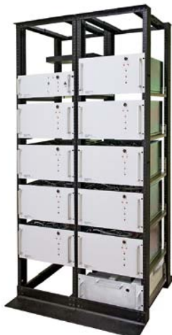
Fig. 2. Set of rack mounted PS5144K and PS5144I units
