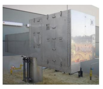
Incorporating high performance thermal insulation materials encapsulated by stainless steel skins, Darshield<sup>™</sup> is supplied in pre-fabricated panel form for assembly and installation onsite or in the factory. Forming a rigid PFP enclosure, the panels are held together using bolts and captive nuts, with the final construction providing the necessary structural integrity to withstand the specified fire and blast conditions.
