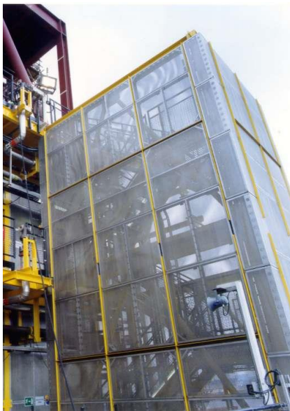
Darscreen™ wind / heat shield protection for escape stair tower
