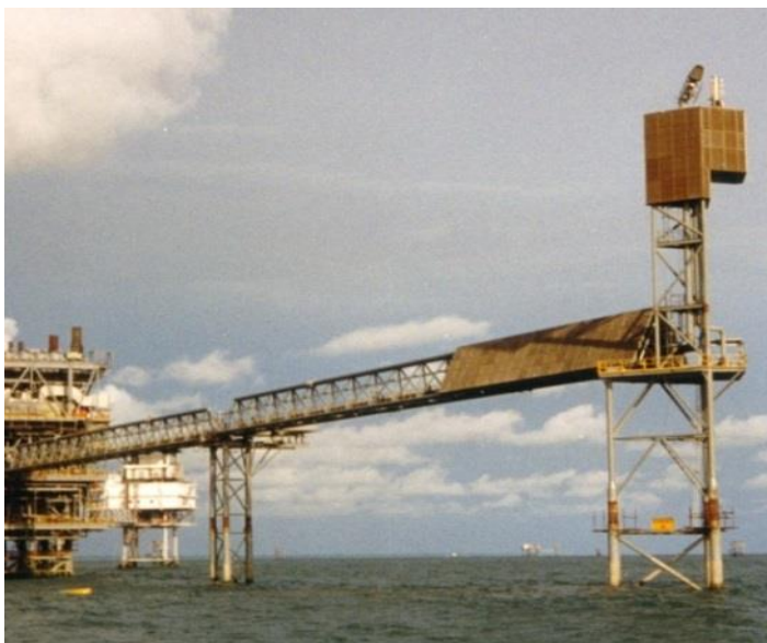
Darscreen™ Woven Mesh system installed on the Escravos Platform, Nigeria
