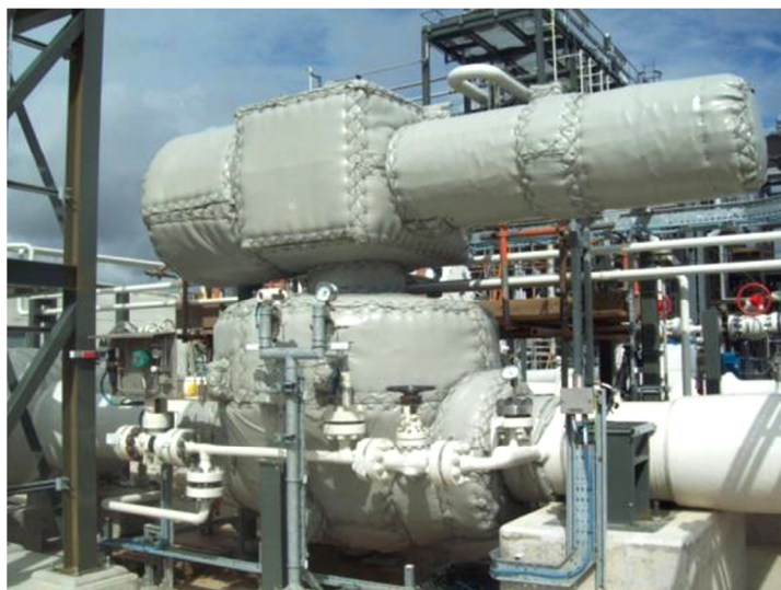
Valves and actuators
