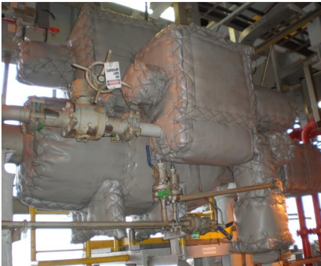
Valves, actuators, and instrumentation
