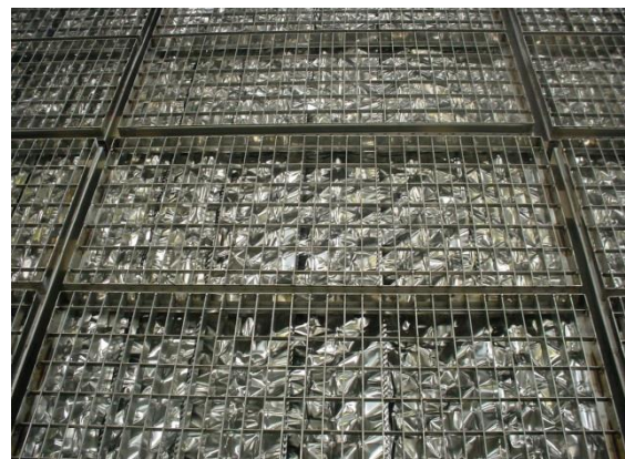
Completed panel sections incorporating grating and foils
