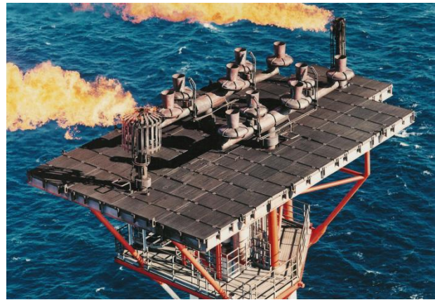
Darflare™ Chevron System installed on BP Bruce, UK North Sea
