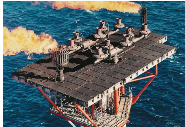
Darflare™ Chevron System installed on BP Bruce, UK North Sea
