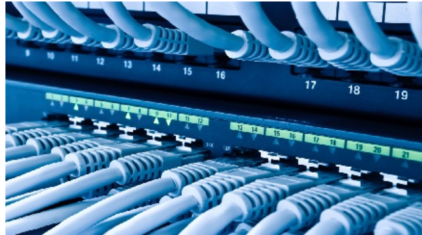
High End Telecom
