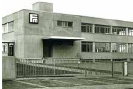
NEUBAU IN HERRENBERG, 1971 NEW CONSTRUCTION IN HERRENBERG, 1971
