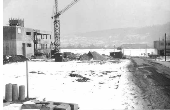
WINTERLICHE BAUSTELLE, 1970 WINTRY CONSTRUCTION SITE, 1970
