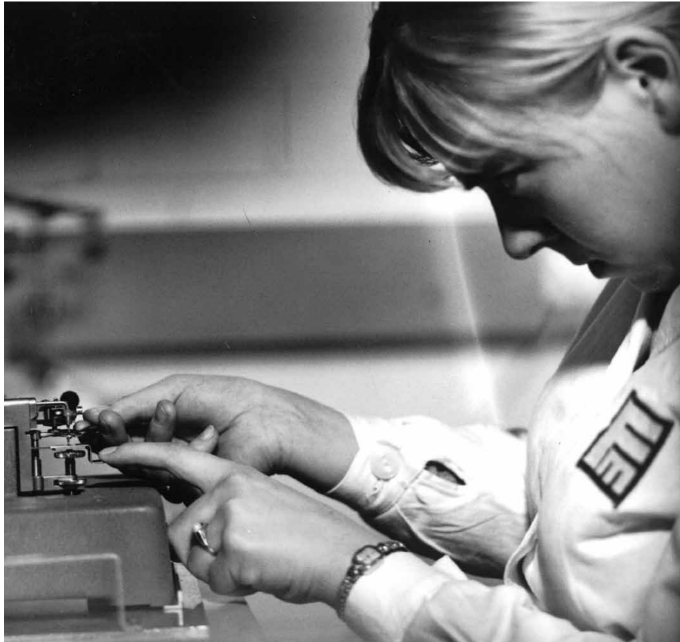
MONTAGE KELVIN-NADELTRÄGER, 1979 ASSEMBLY OF KELVIN NEEDLE CARRIERS, 1979
