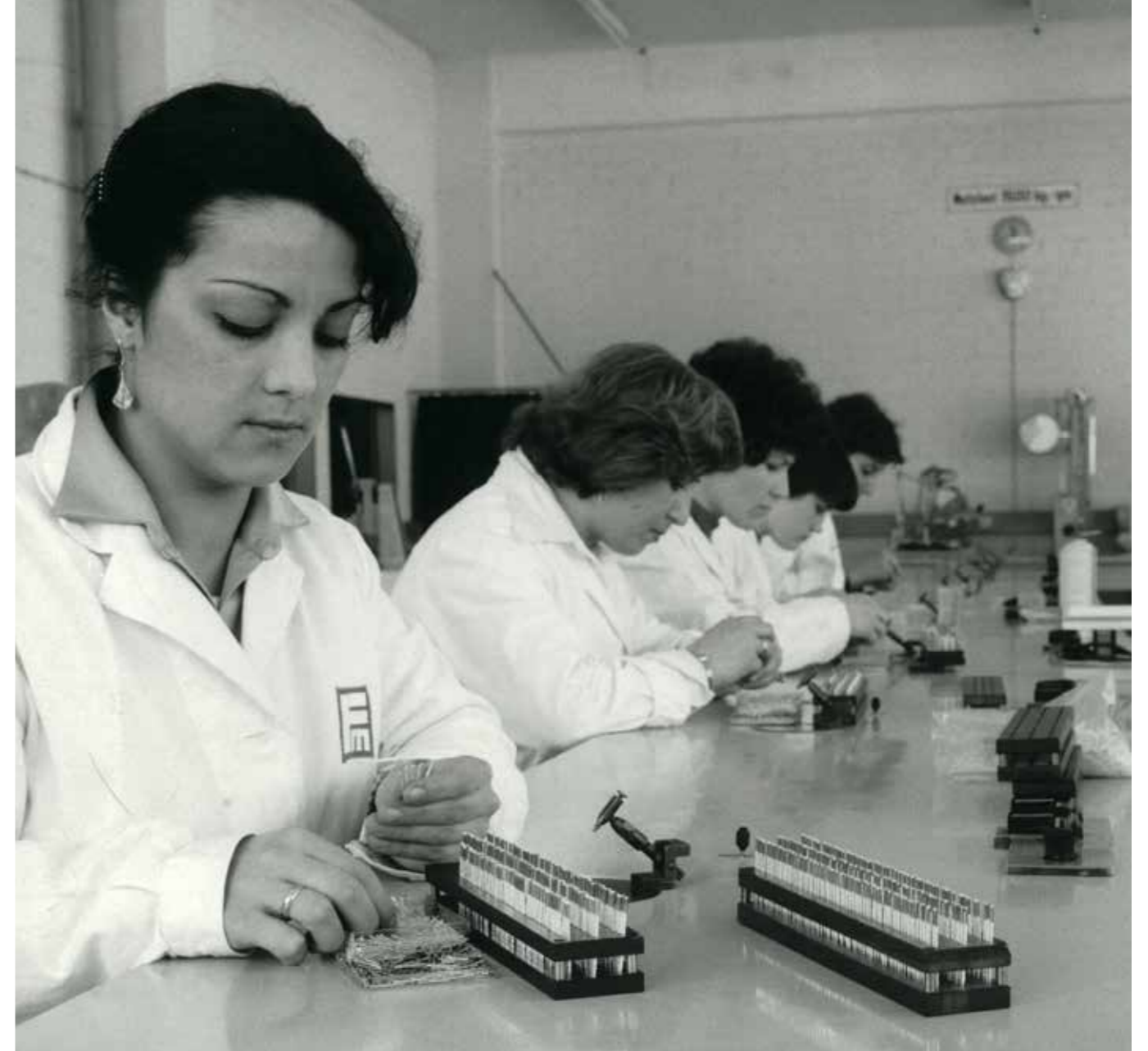
MONTAGE VON FEDERKONTAKTSTIFTEN, 1974 ASSEMBLY OF SPRING CONTACT PROBES, 1974
