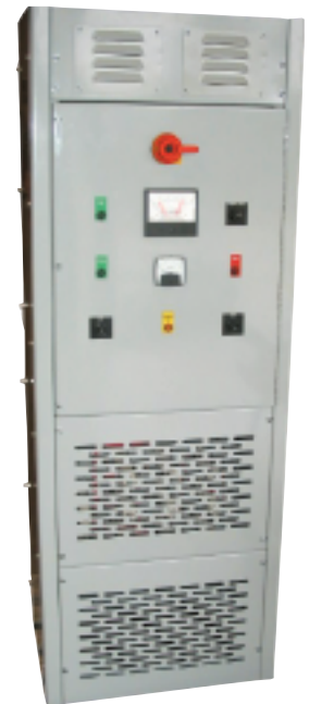
High Resistance Grounding System
